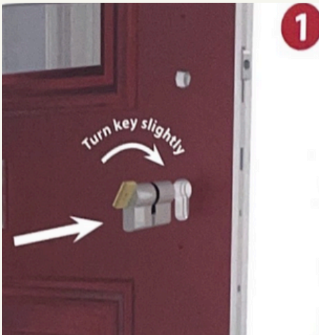
1. Insert cylinder and turn the key slightly
