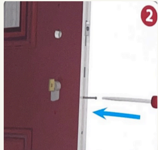
2. Insert screw and tighten
